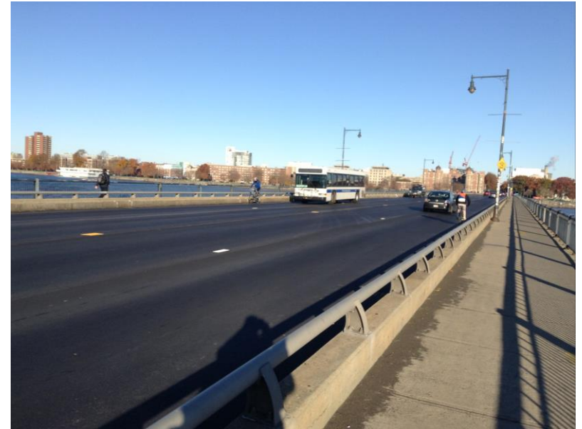
Changes to road surface
