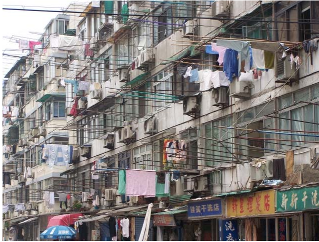
Shànghǎi jūmínlóu ('residential building'). [JKW 2006]
