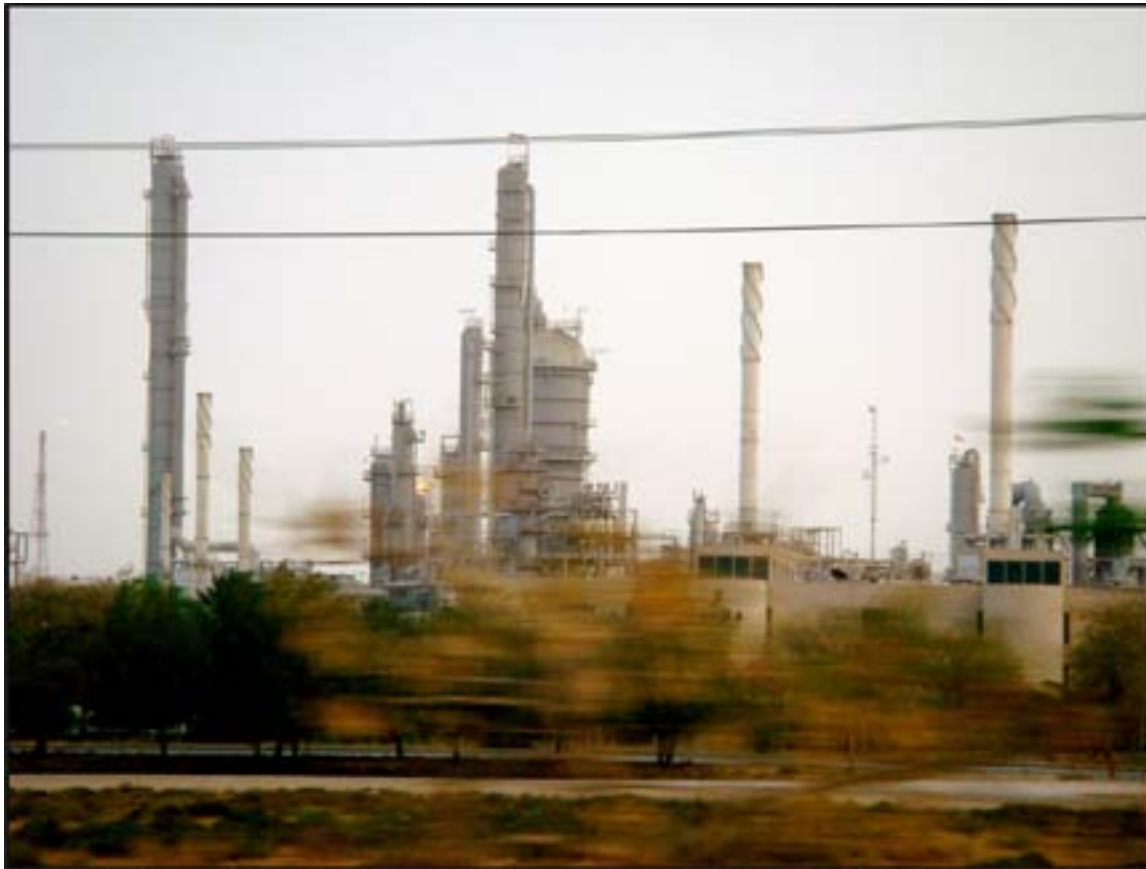
Jubail Desalination Plant
